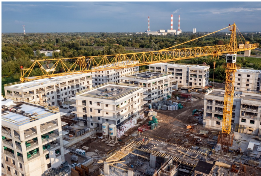
Construction in Warsaw, Poland
