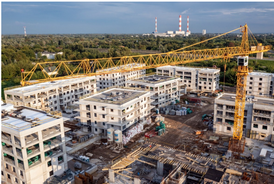
Construction in Warsaw, Poland
