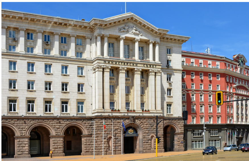
Council of Ministers building, Sofia
