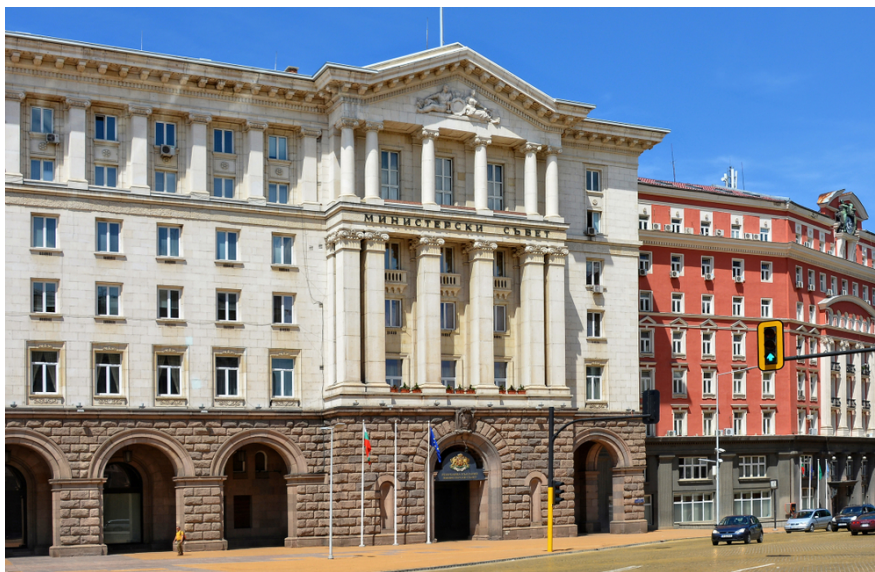
Council of Ministers building, Sofia
