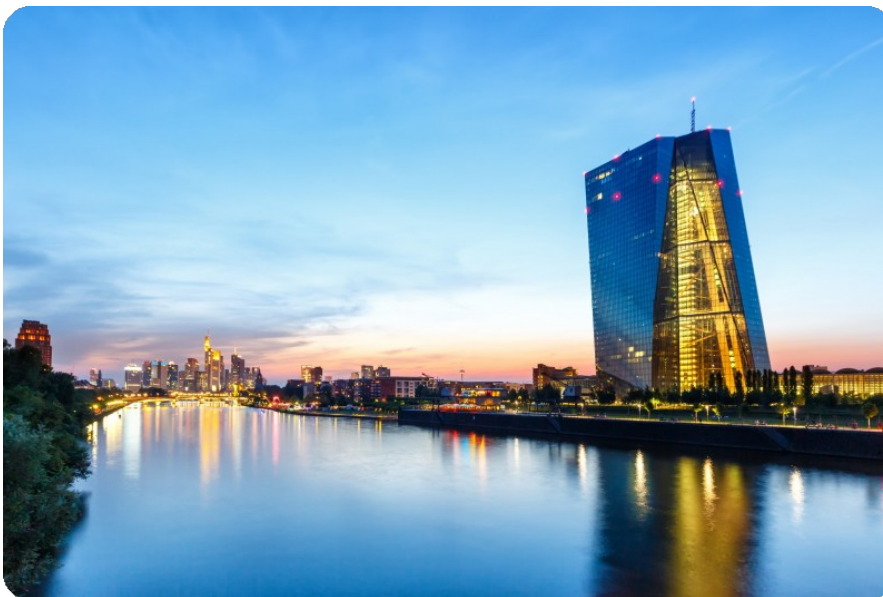
European Central Bank building and the Frankfurt skyline
