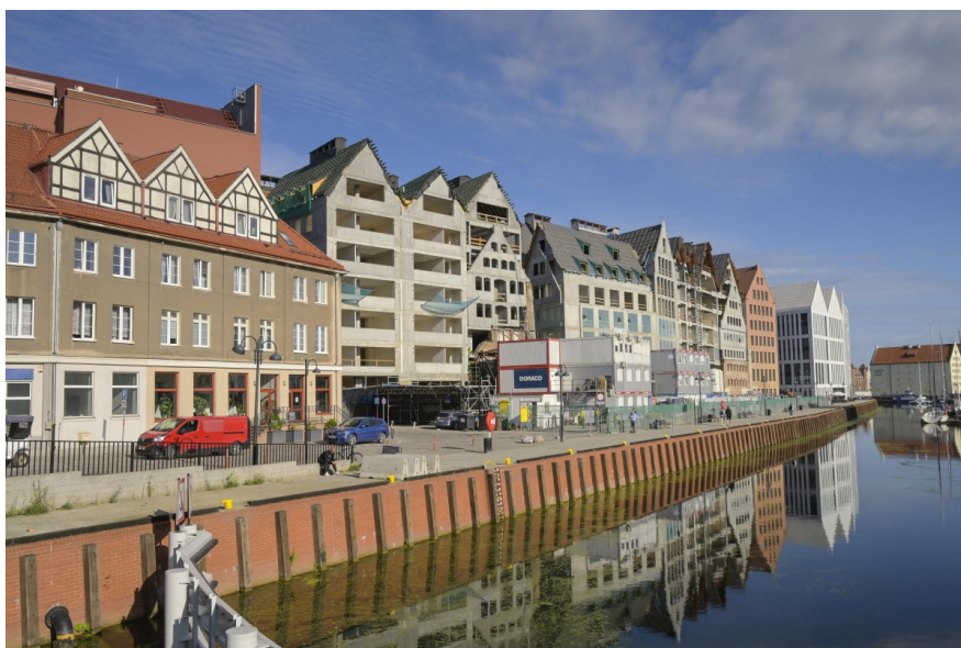
New housing construction in Gdańsk, Poland
