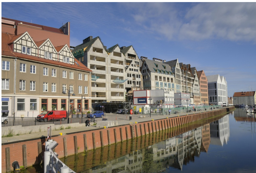
New housing construction in Gdańsk, Poland
