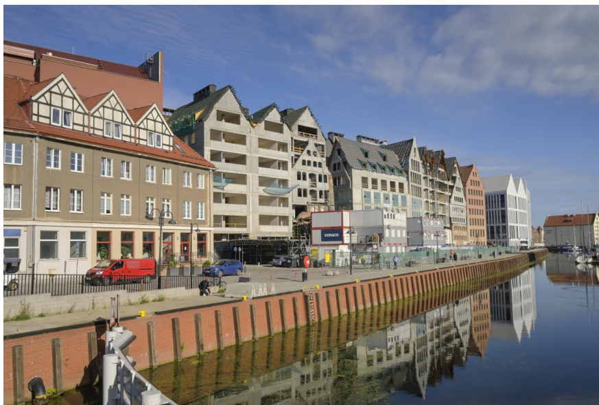
New housing construction in Gdańsk, Poland
