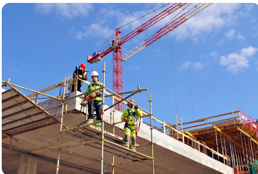
Construction workers in Warsaw, Poland
