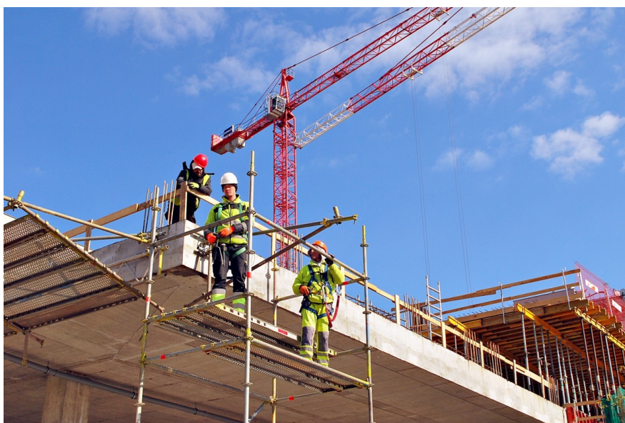
Construction workers in Warsaw, Poland
