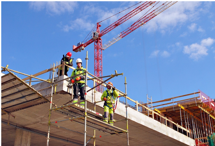
Construction workers in Warsaw, Poland
