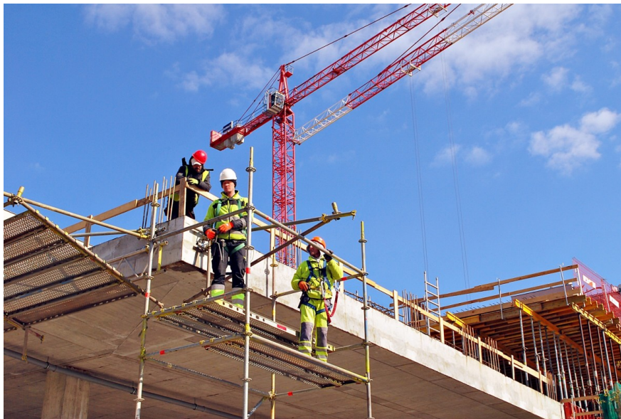
Construction workers in Warsaw, Poland
