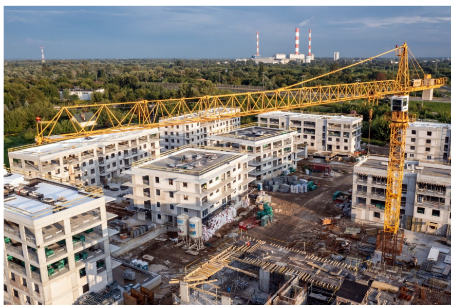
Construction in Warsaw, Poland
