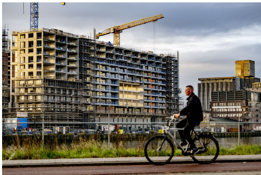
New homes under construction in Rotterdam, the Netherlands
