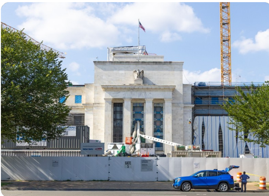
The US Federal Reserve, currently under construction
