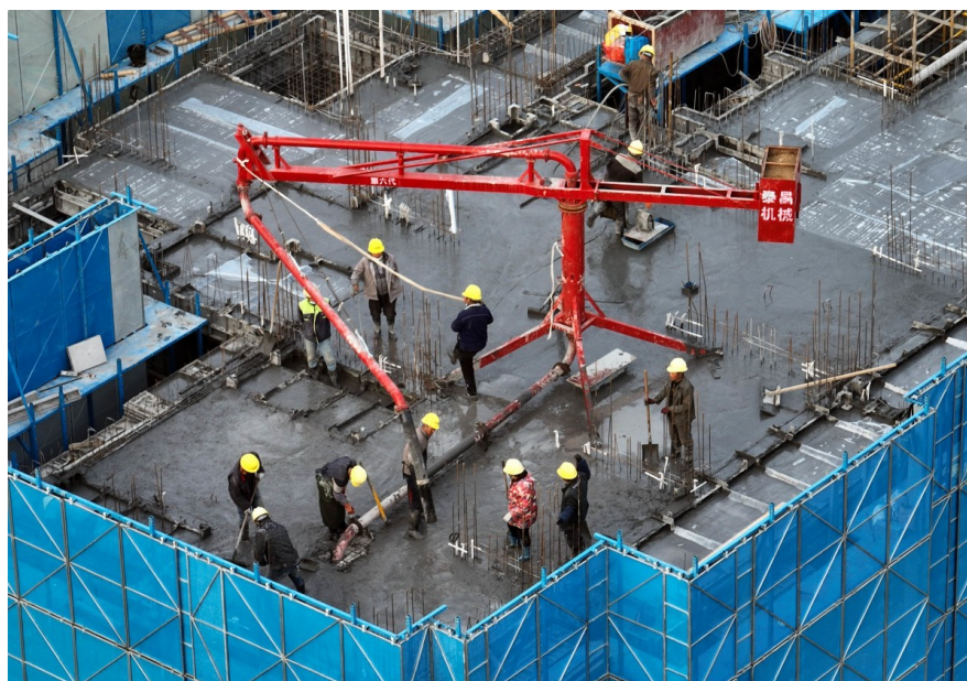
Real estate continues to be a drag on China's economy. Pictured: a residential construction site in Huaian, eastern China
