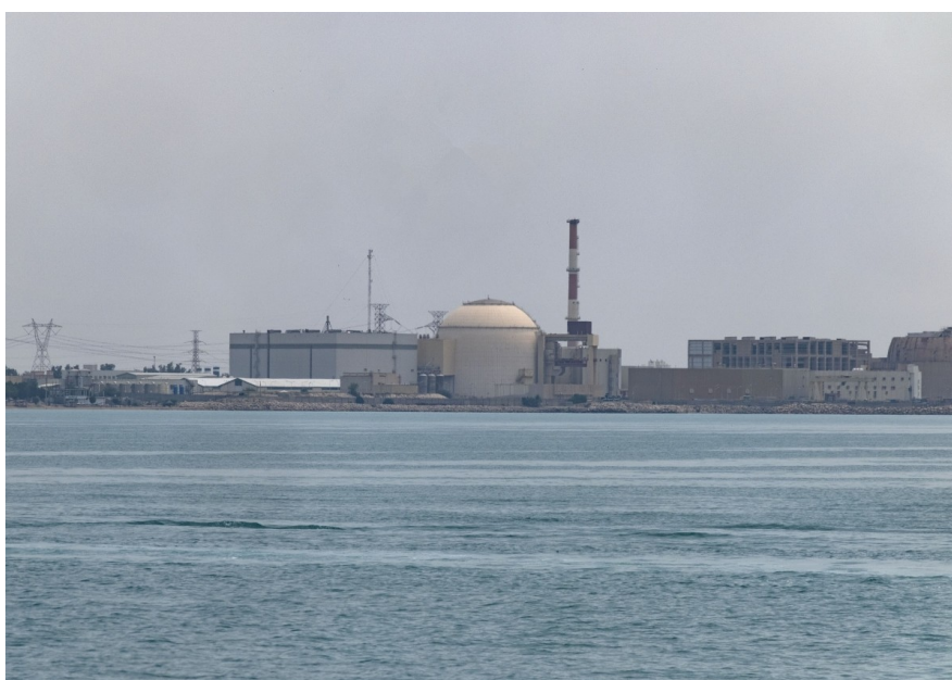
Bushehr nuclear power plant in Iran
