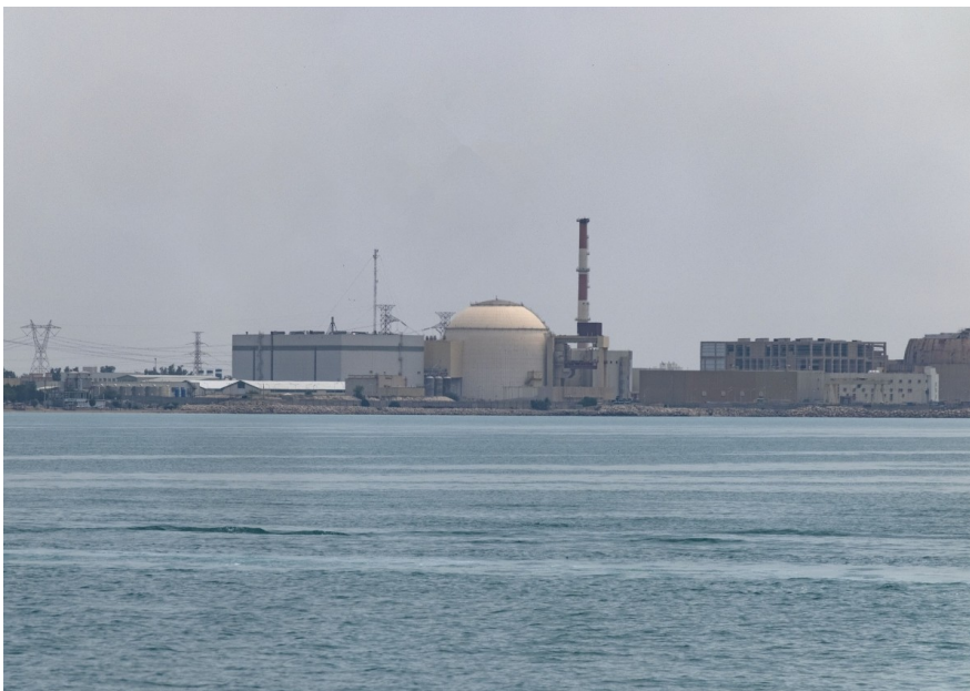
Bushehr nuclear power plant in Iran
