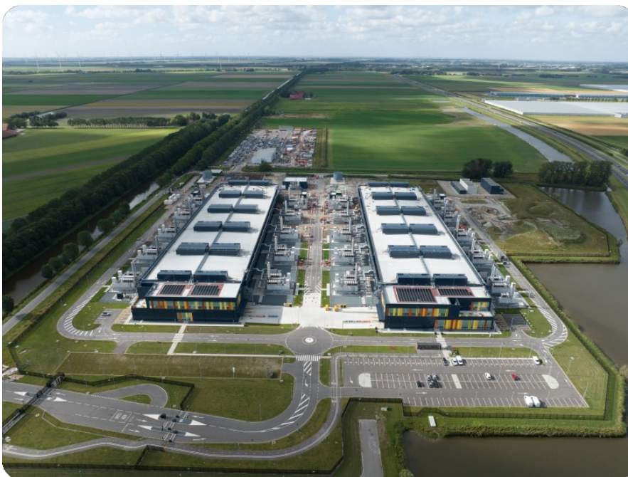
A data centre in the Netherlands
