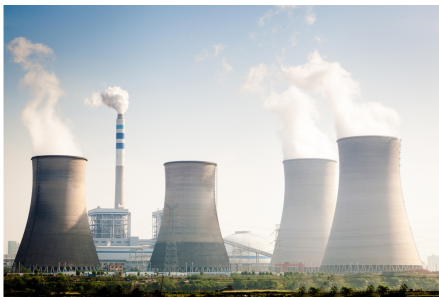
A nuclear power plant Dukovany, Czech Republic
