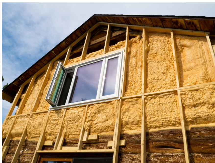
Renovation of an old home with energy efficient insulation and windows
