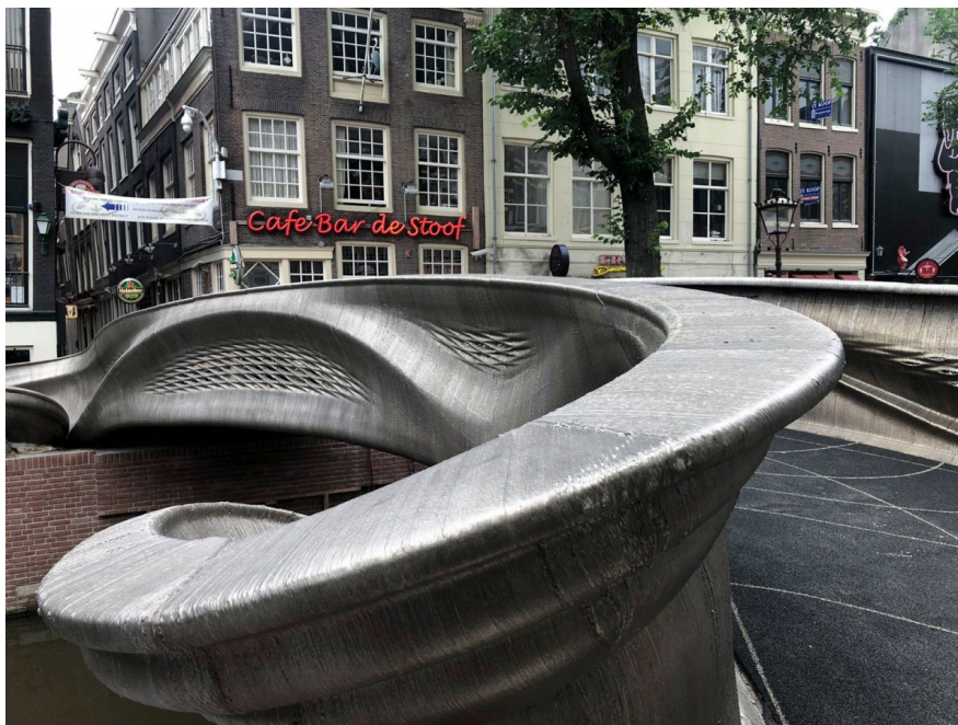
This 3D printed pedestrian bridge, recently opened in Amsterdam, shows that the technology is well-suited to making complex shapes
