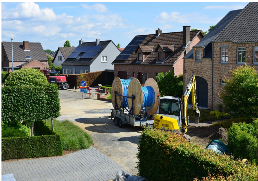
Leuven, Flemish-Brabant, Belgium: installation of telecom fiber optic, June 2024
