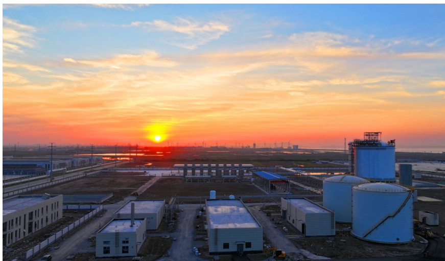
LNG storage and distribution station project in Lianyungang City, China
