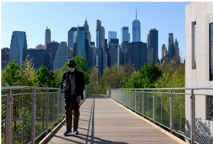
People walk on Brooklyn Bridge Park's rebuilt Squibb Bridge in New York.
