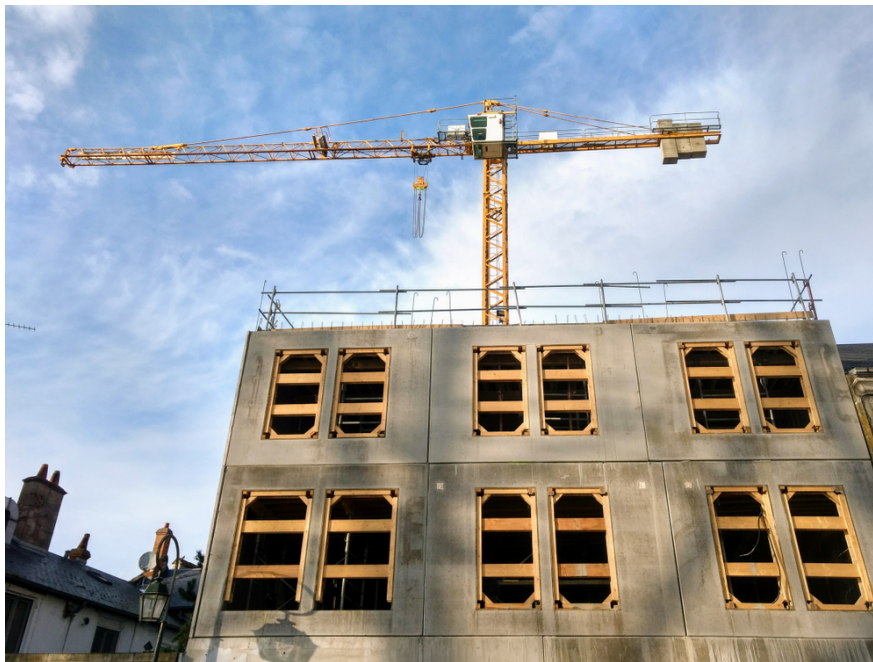
House construction in Orleans, France
