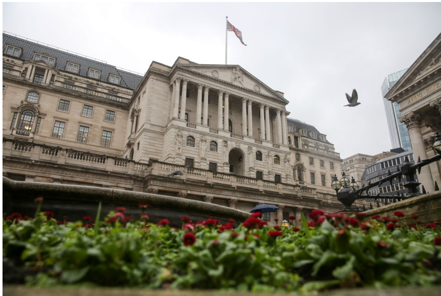
The Bank of England in the City of London, UK
