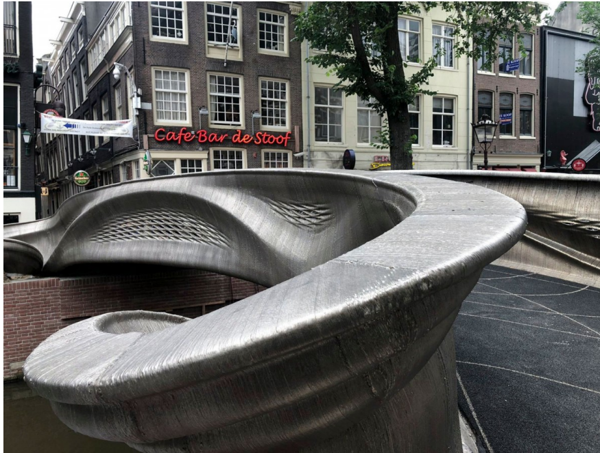
This 3D printed pedestrian bridge, recently opened in Amsterdam, shows that the technology is well-suited to making complex shapes
