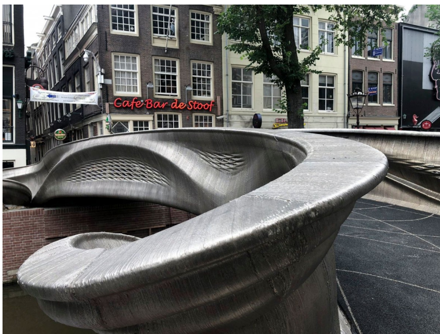
This 3D printed pedestrian bridge, recently opened in Amsterdam, shows that the technology is well-suited to making complex shapes
