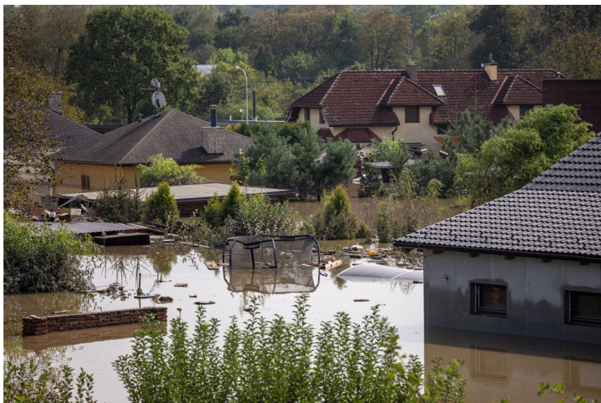
Houses in a flood-affected area following heavy rain in the town of Ostrava, Czechia
