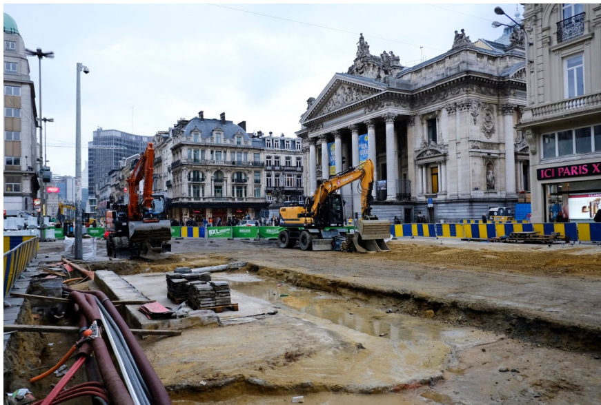
Street construction in central Brussels
