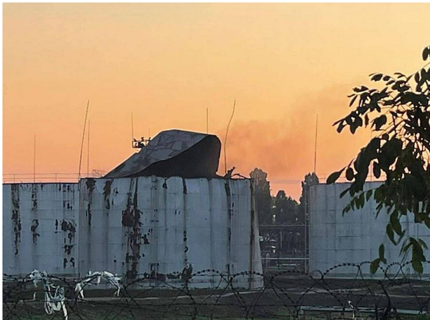
An image released by the Ukrainian military said to show a damaged port infrastructure on the Danube River in the Odesa region
