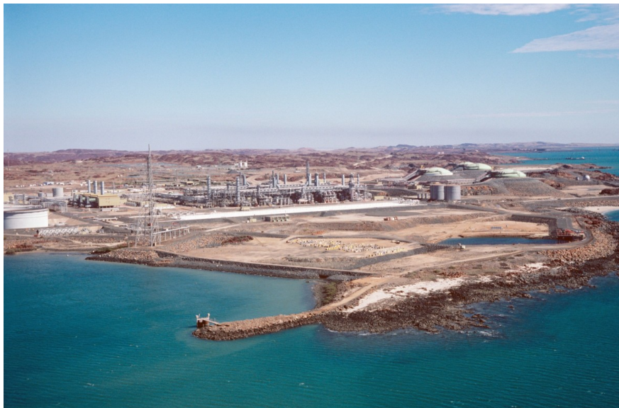
Australia's North West Shelf gas plant
