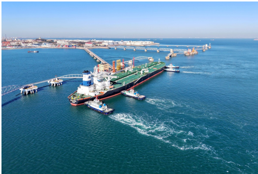
A foreign oil tanker prepares to leave the dock after unloading crude oil at the port of Qingdao in the Shandong province, China
