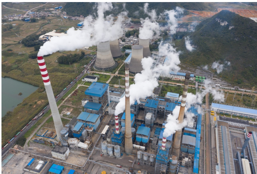
A large aluminium ore processing plant in China
