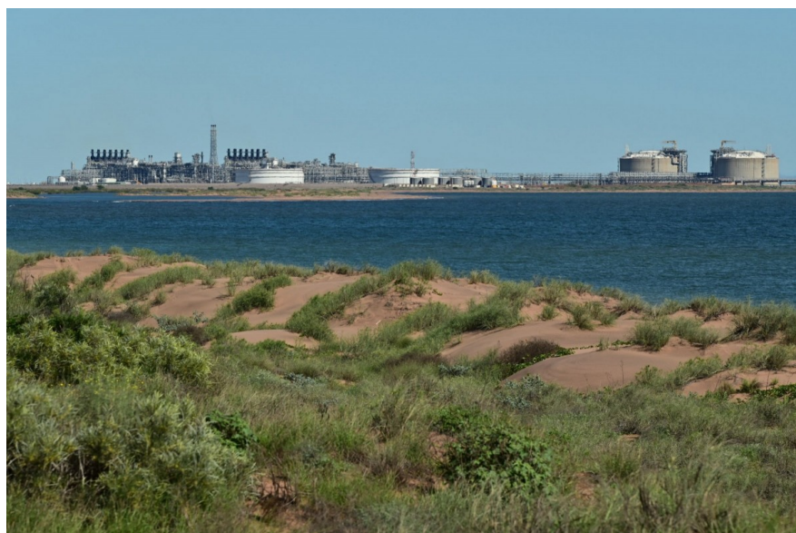
Unions in Australia have served a strike notice to Chevron for workers at its Wheatstone LNG operations (pictured)
