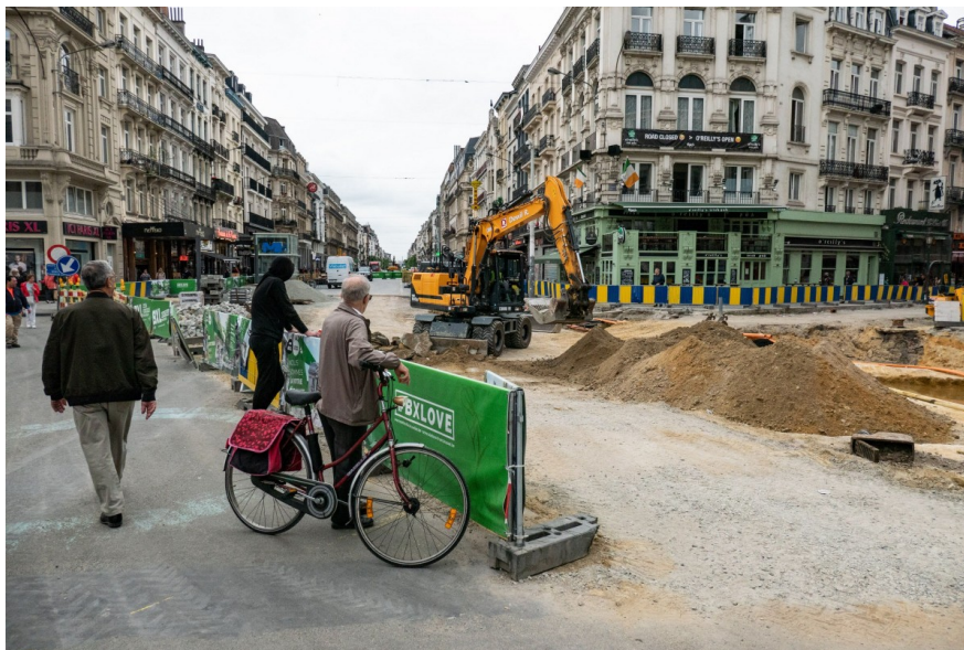
Construction work in the centre of Brussels, Belgium
