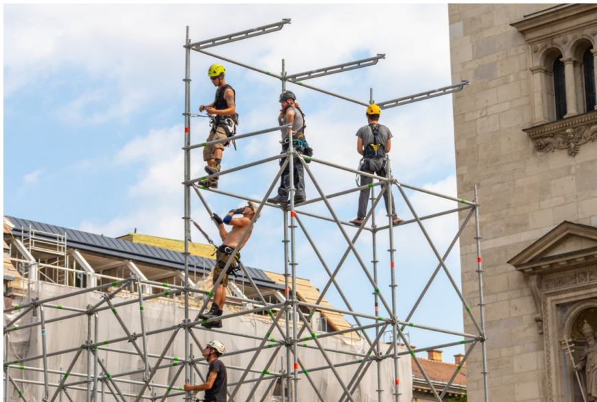
Construction workers in Budapest, Hungary
