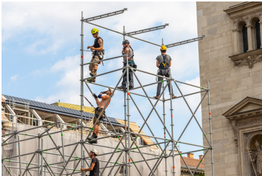
Construction workers in Budapest, Hungary
