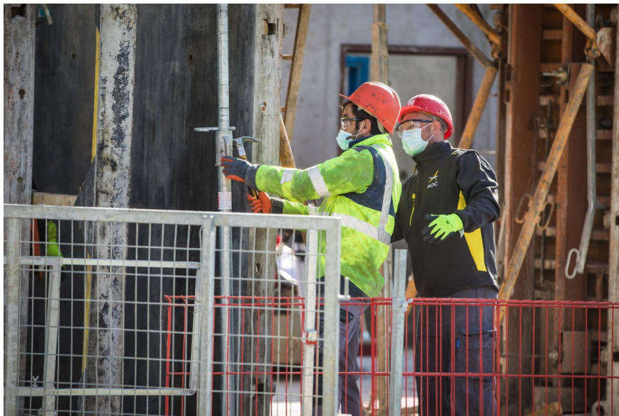
Construction workers on a building site in France
