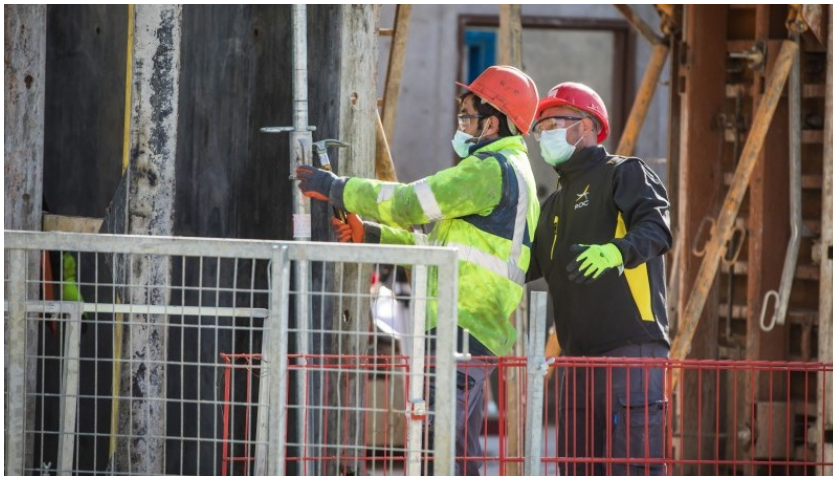
Construction workers on a building site in France
