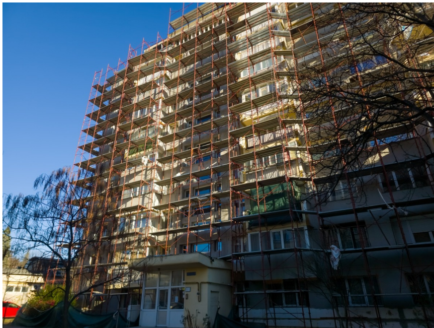
A building renovation in Piatra Neamt, Romania
