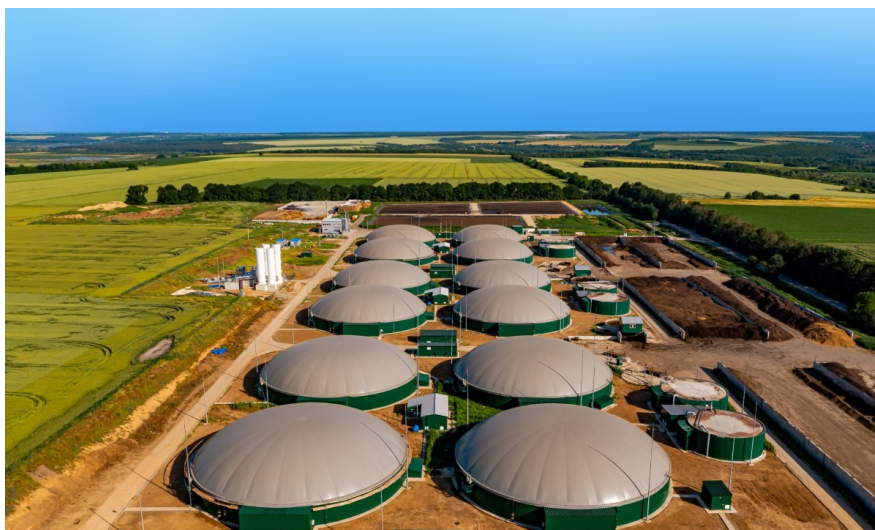
Biogas plants convert organic waste like agricultural residue, manure, and food scraps into biogas, which is then refined into RNG
