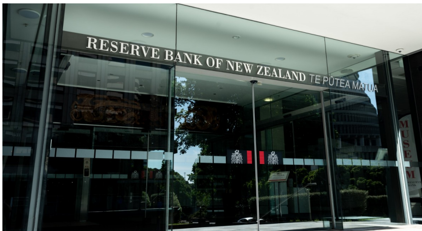
Reserve Bank of New Zealand building
