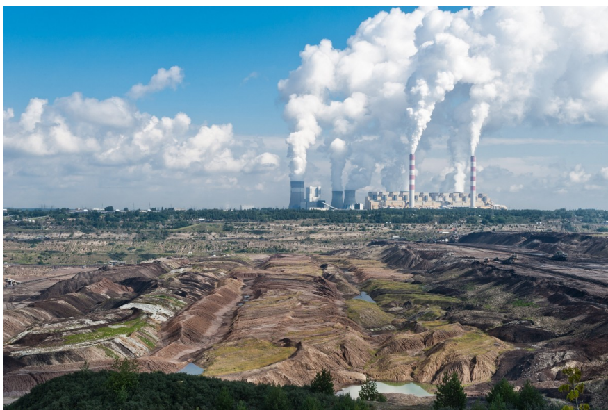
Coal power plant in Bełchatów, Poland
