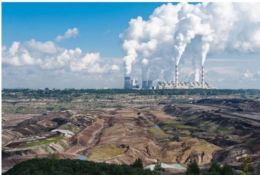
Coal power plant in Bełchatów, Poland
