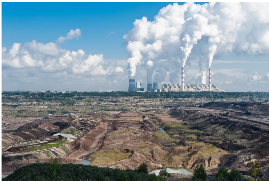
Coal power plant in Bełchatów, Poland
