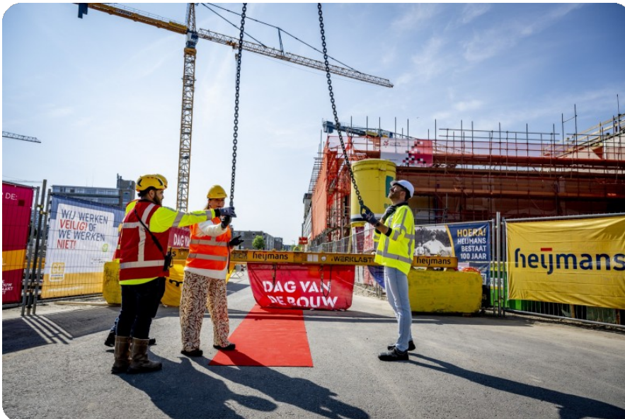
A construction site in Rotterdam, the Netherlands
