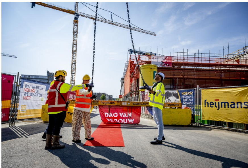
A construction site in Rotterdam, the Netherlands
