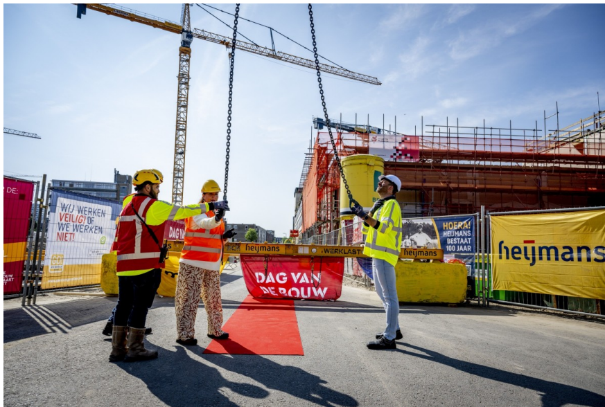
A construction site in Rotterdam, the Netherlands
