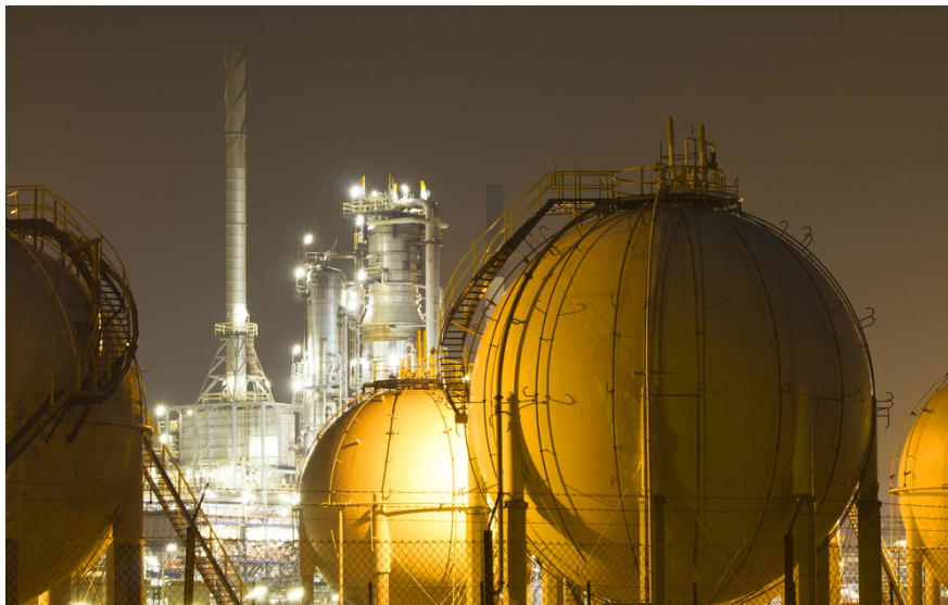
Gas storage tank
