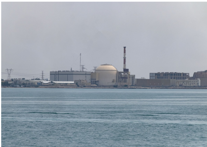
Bushehr nuclear power plant in Iran
