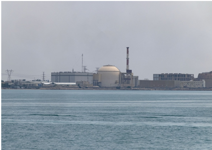
Bushehr nuclear power plant in Iran
