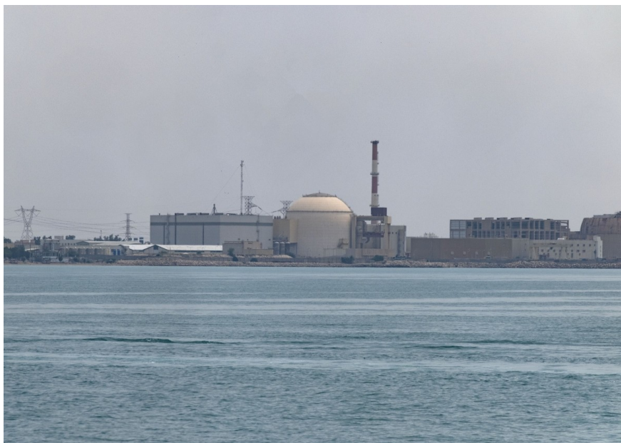
Bushehr nuclear power plant in Iran
