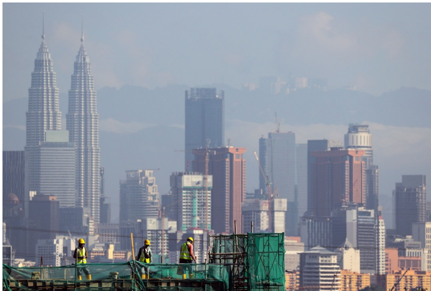
Workers labour on scaffolding at a construction site in Kuala Lumpur
