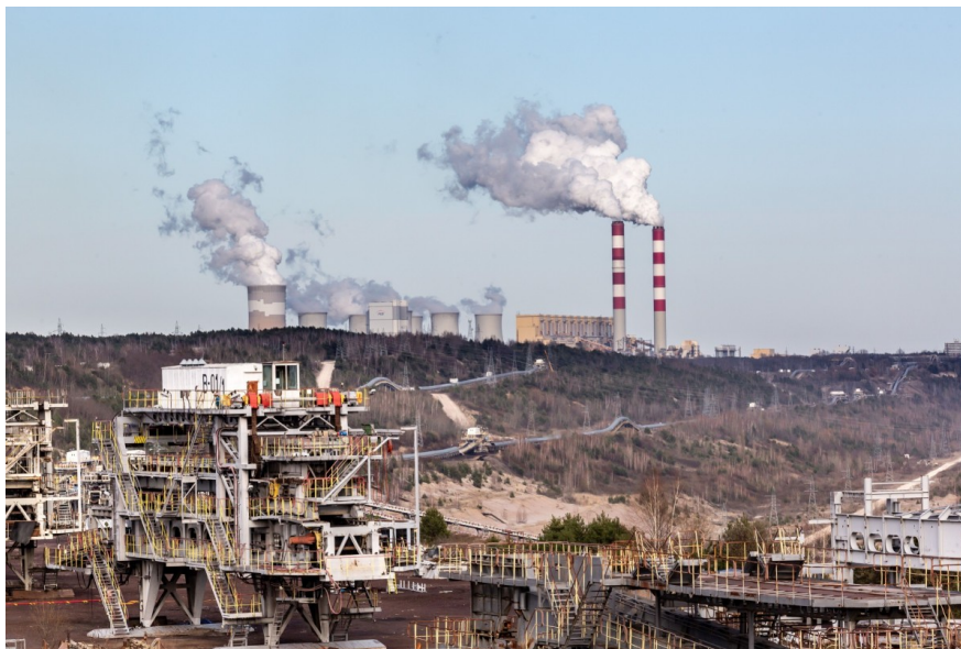
Bełchatów Power Station, the largest coal power plant in Poland
