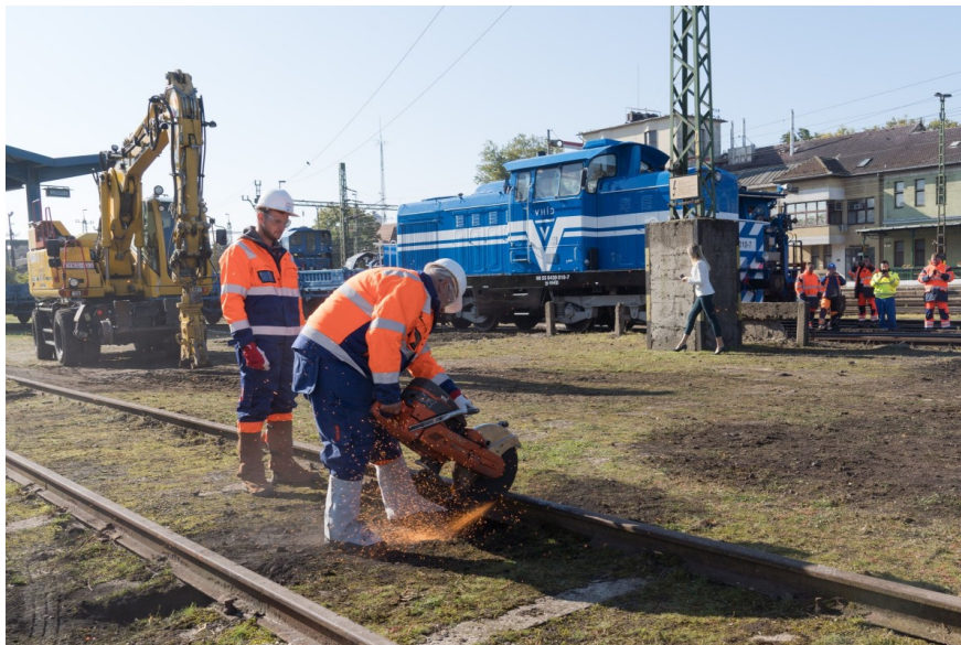
Workers at the the Budapest-Belgrade railway in Kiskunhalas, Hungary
