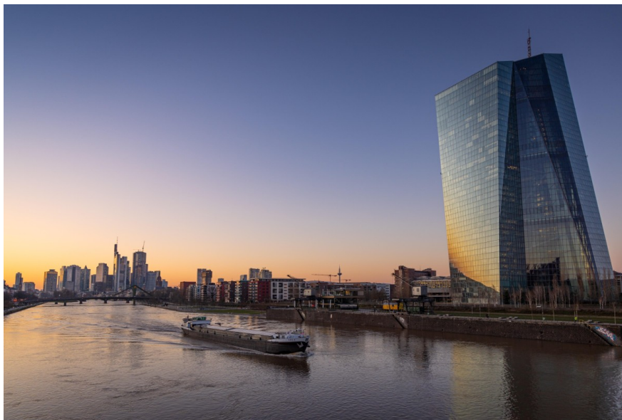
The European Central Bank's main building in Frankfurt, Germany
