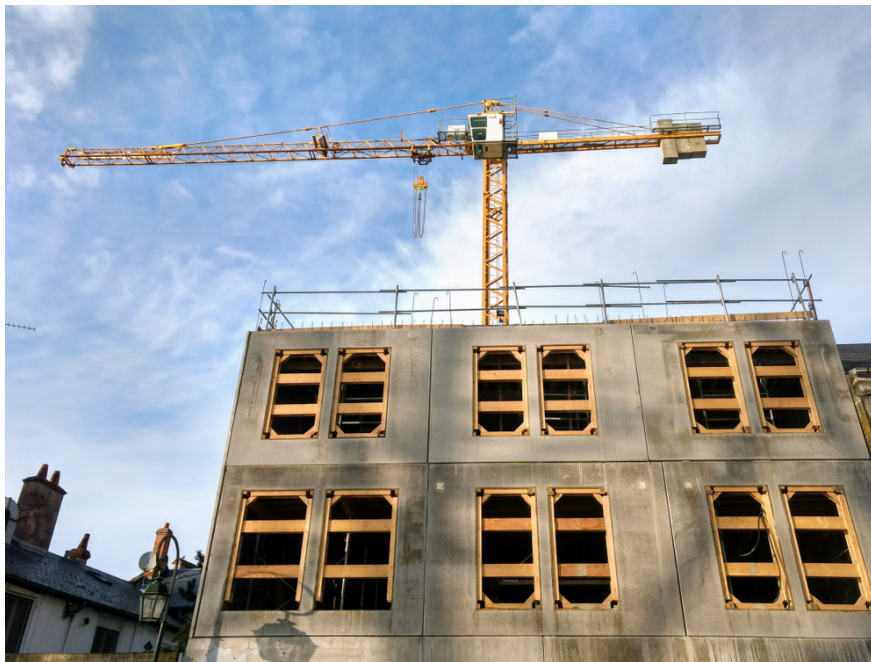
House construction in Orleans, France
