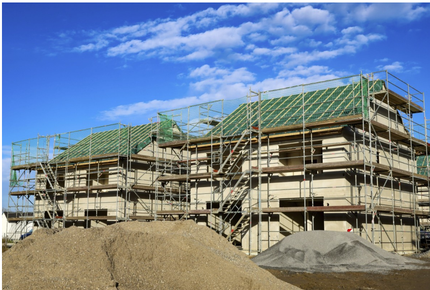
Energy-efficient homes being built in North Rhine-Westphalia, Germany
