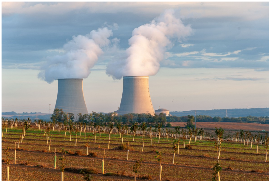
Nuclear power plant Nogent-sur-Seine, France
