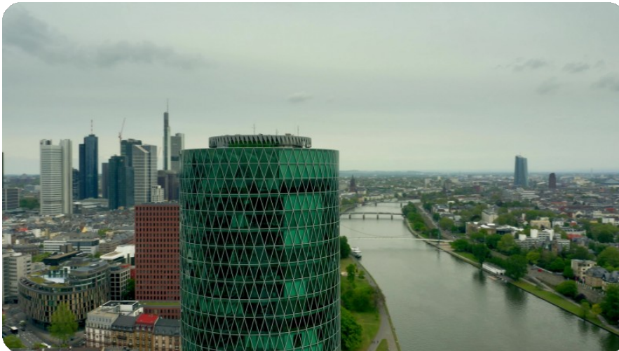
Aerial shot of the European Insurance and Occupational Pensions Authority headquarters in Frankfurt, Germany
