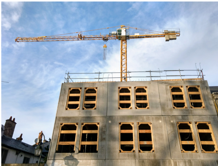
House construction in Orleans, France
