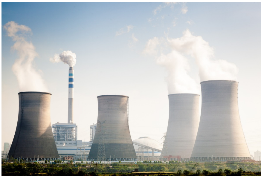
A nuclear power plant Dukovany, Czech Republic
