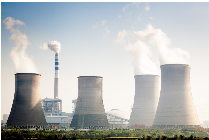
A nuclear power plant Dukovany, Czech Republic
