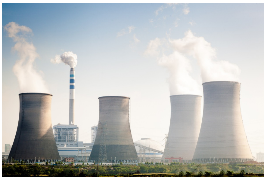
A nuclear power plant Dukovany, Czech Republic
