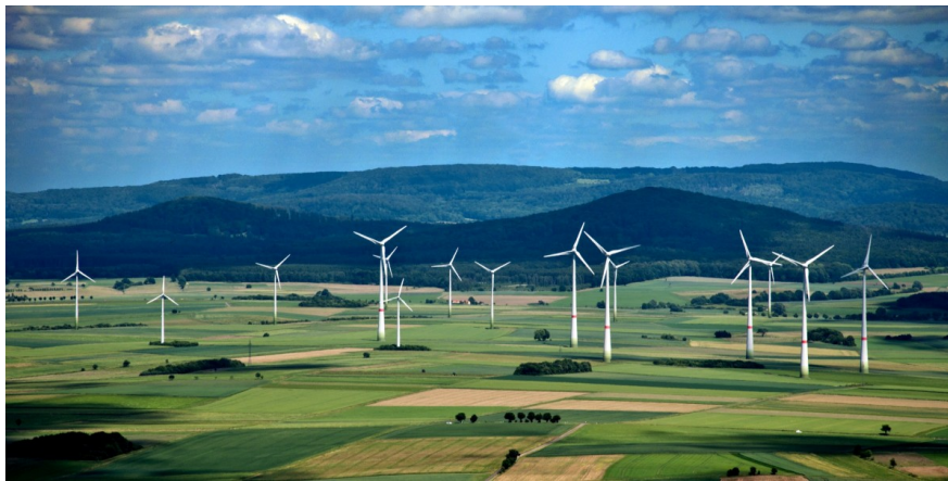
A wind farm in Hesse, Germany
