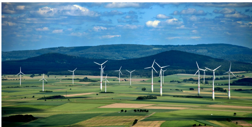
A wind farm in Hesse, Germany
